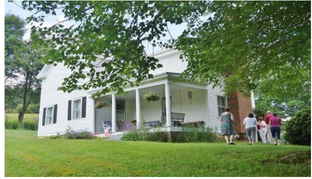
Christopher Slusher Jr. homeplace on Laurel Branch Rd.
